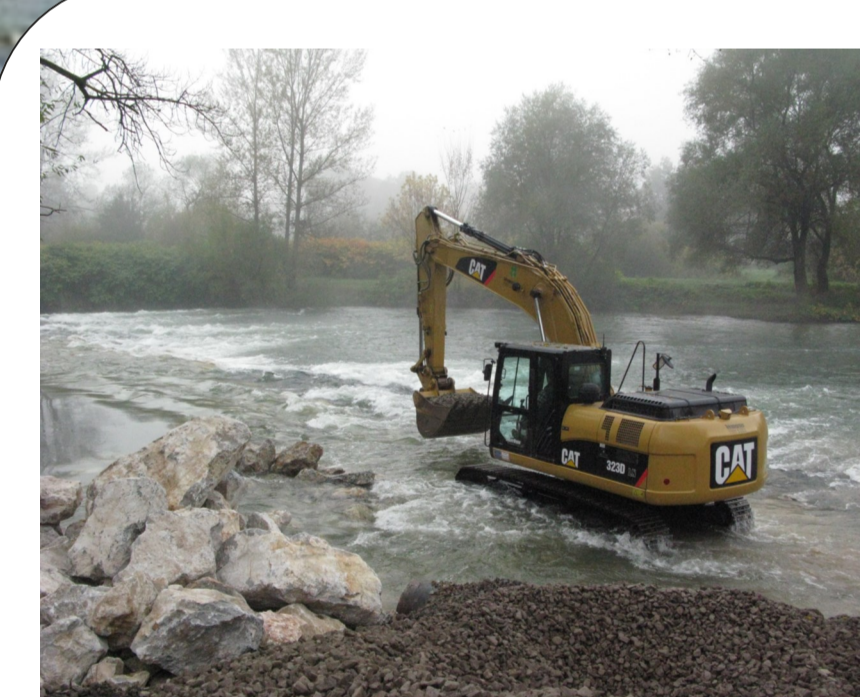
Reconstruction of the sill
