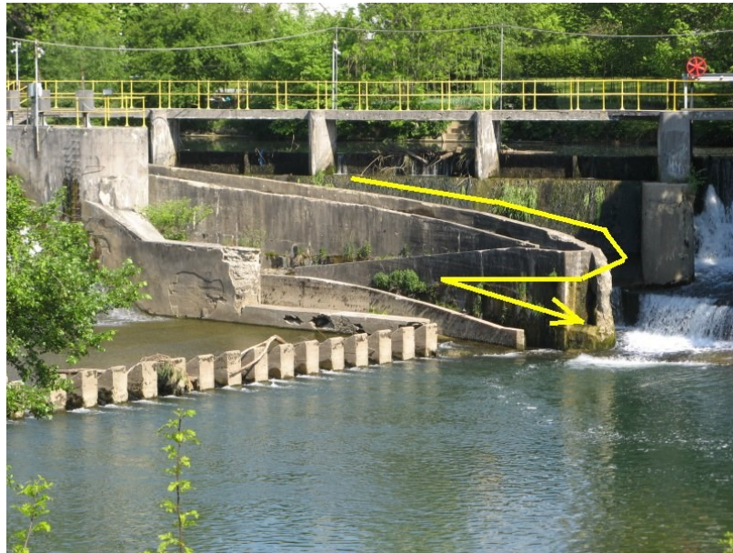
Figure 2: Fish pass at the Fužine weir
