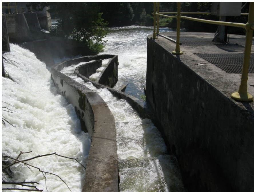
Figure 3: Fish pass at the Fužine weir
