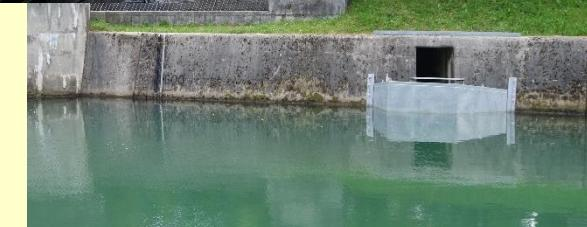
Element for preventing accumulation of floating debris
