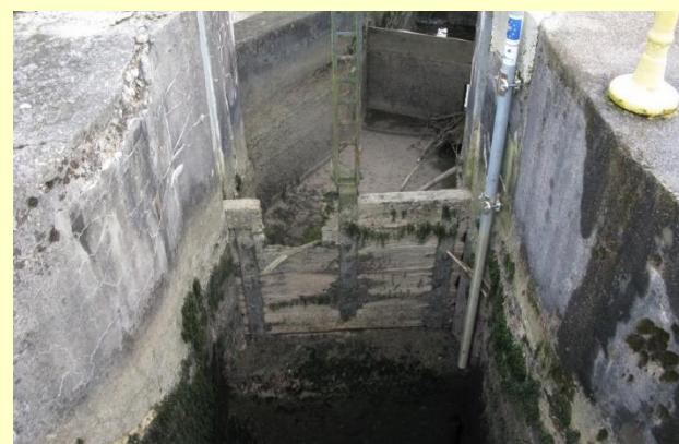
Fish pass has collapsed during the high flow in November 2013
