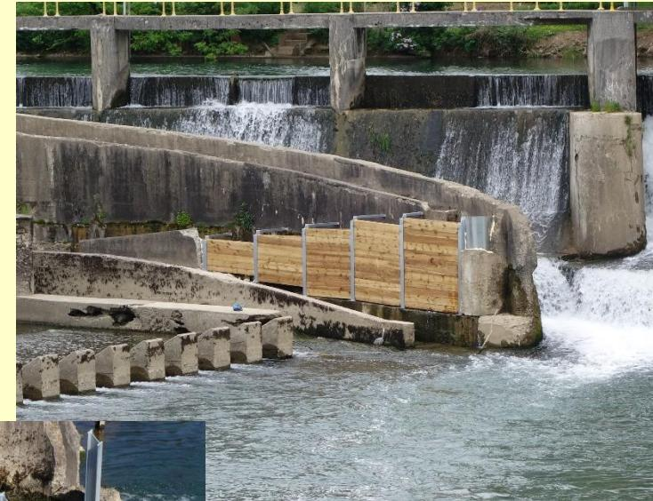
The collapsed part of fish pass was reconstructed using steel pylons filled with wood wall
