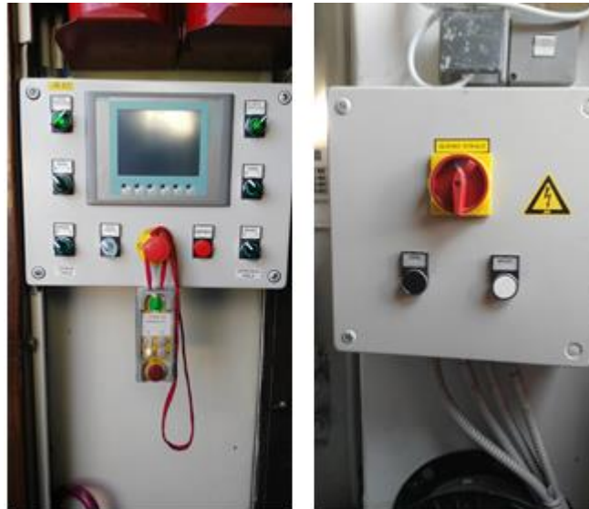
Figure 4: Touch screen indicating the position of the gate (left) and the main switchboard (junction box) (right)
