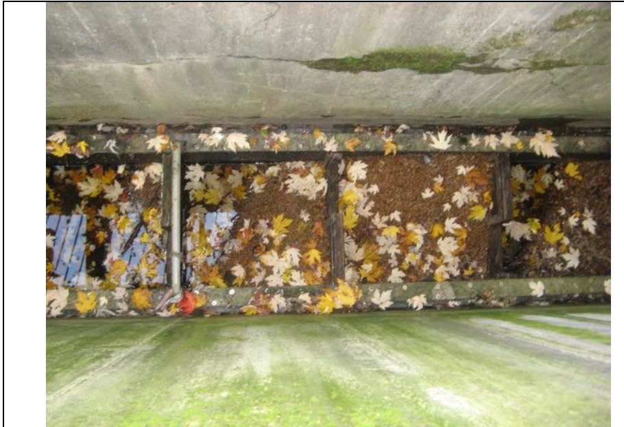
Figure: Fish pass on Ambrož weir is dry and no operating when weir is opened, 8.11.2012
