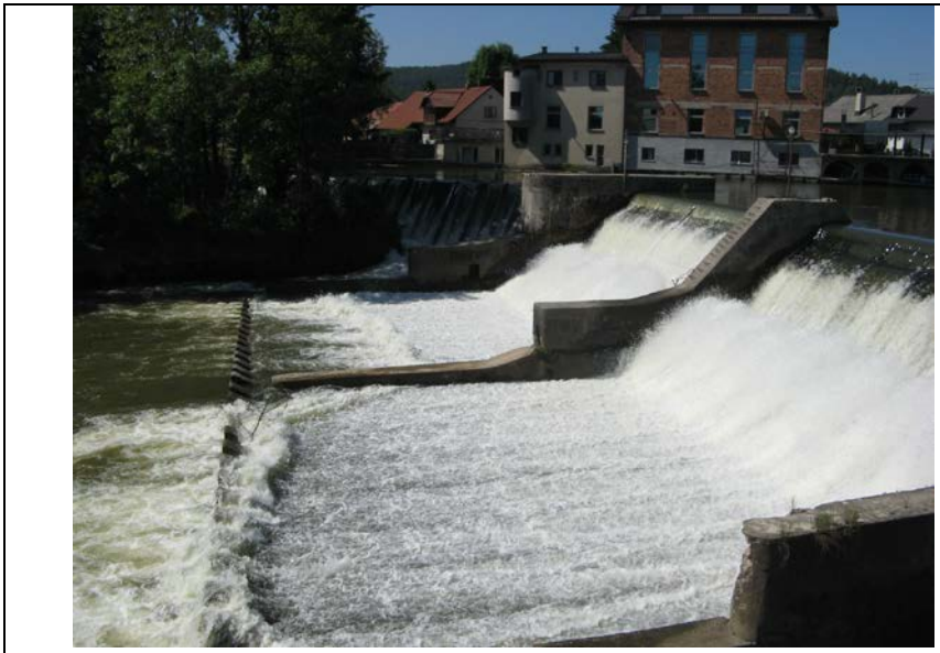
Figure: Fužine weir
