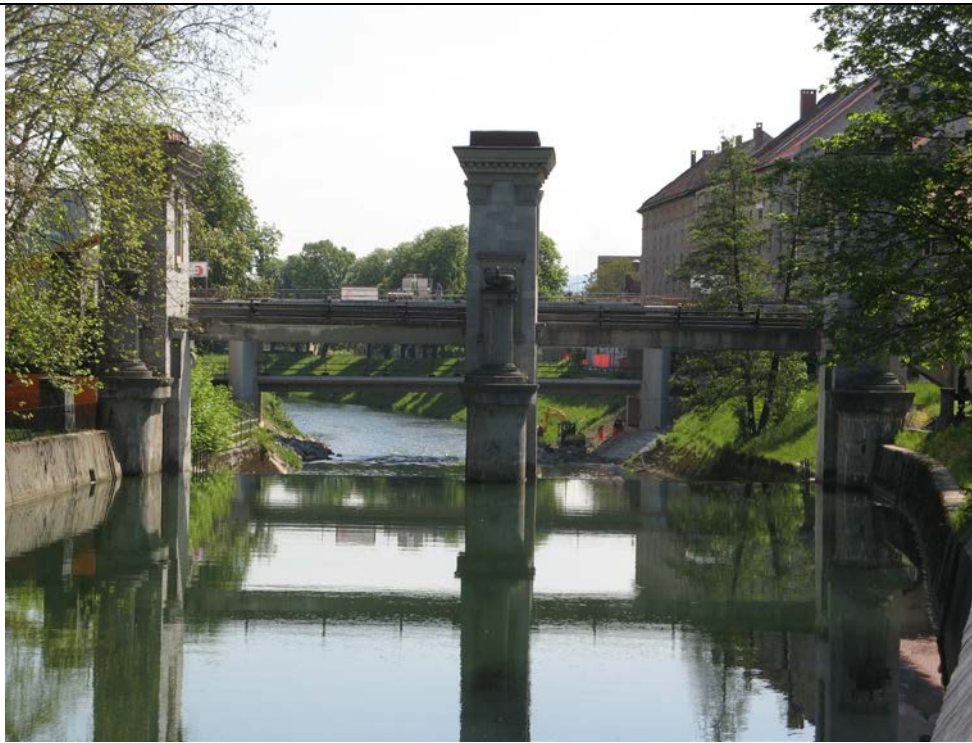
Figure: Weir at Ambrož Square, view from upstream
