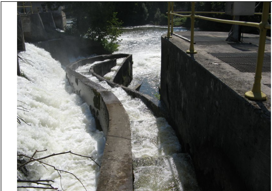
Figure: Degraded old fish pass
