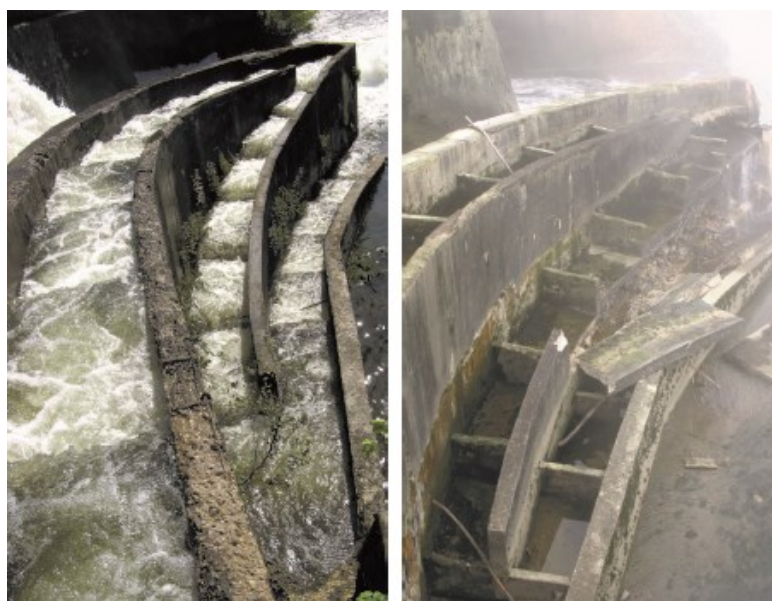
Figure 10: Fish pass on Fužine weir before and after the high flow in November 2013
