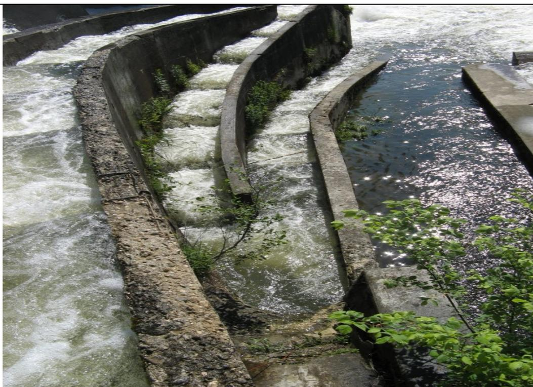
*Figure 07: Downstream fish pass Fužine, 18.5.2012*
