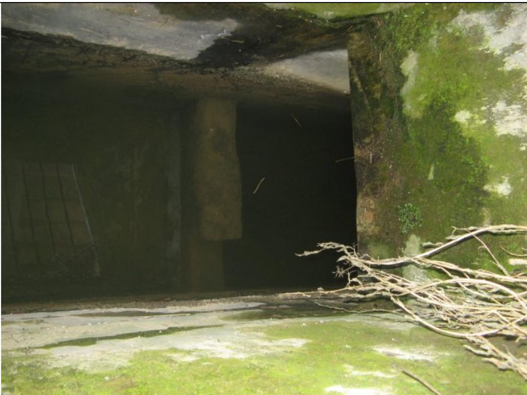
*Figure 24: Fish pass on Ambrož weir, no water flow on downstream side, 8.11.2012*
