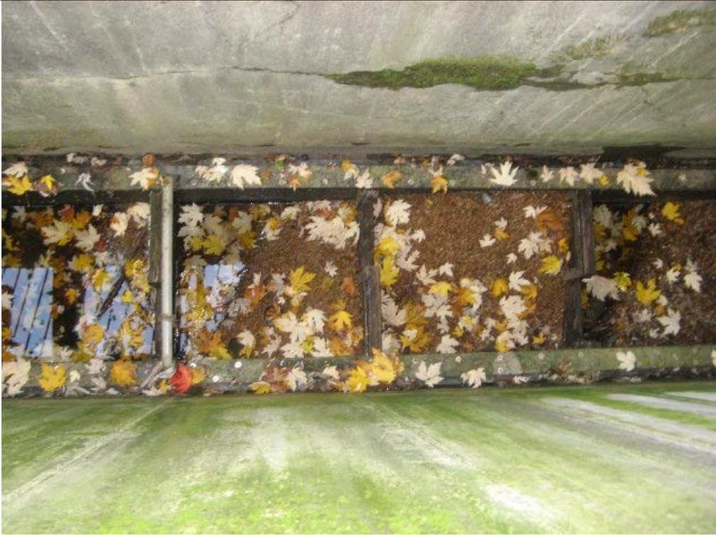
*Figure 23: Fish pass on Ambrož weir is dry and no-operating when weir is opened, 8.11.2012*
