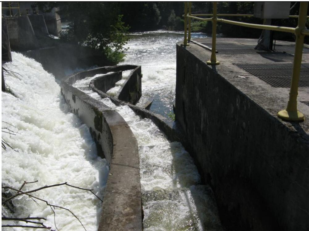
*Figure 16: Degraded old fish pass, 18.5.2012*
