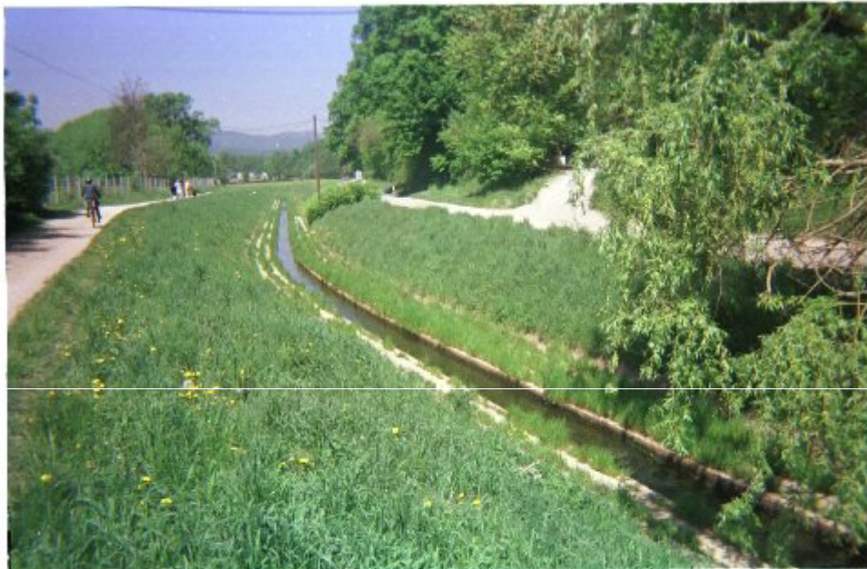
Figure 11. The Glinščica watercourse channel in Ljubljana.
