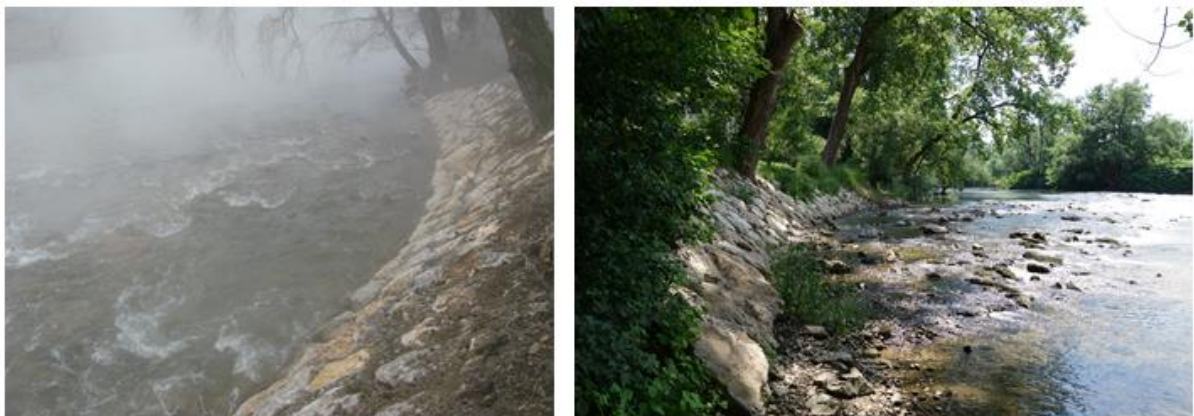
Figure 3: The restored right bank right after the completion of works in October 2013 (left) and in the summer of 2015 (right).
