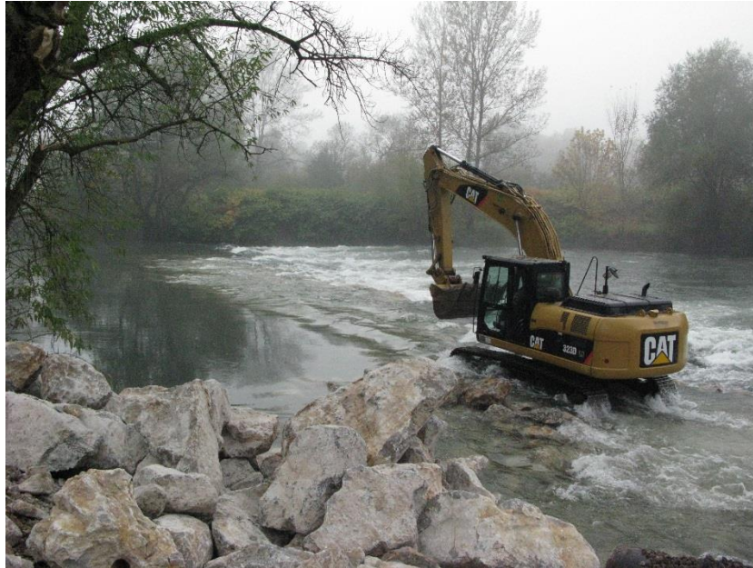
Figure 2: Restoration works for sill stabilisation using a dredger
