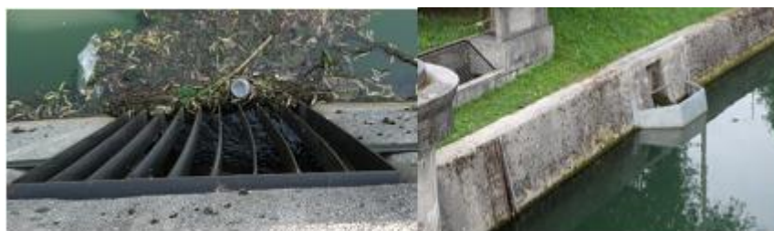
Figure 5: Situation before (left) and after (right) the installation of protection against floating debris at the inflow into the fish pass (Ambrožev trg)
