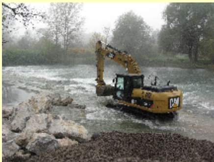
Concrete restoration actions
