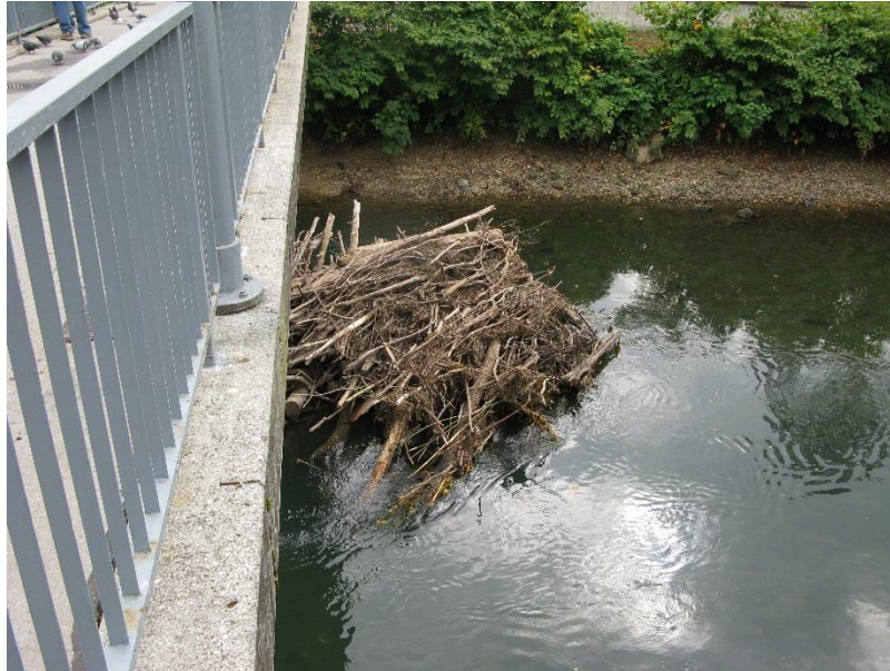
Figure 5: The build-up of debris behind the grill prior to the restoration of the fish pass
