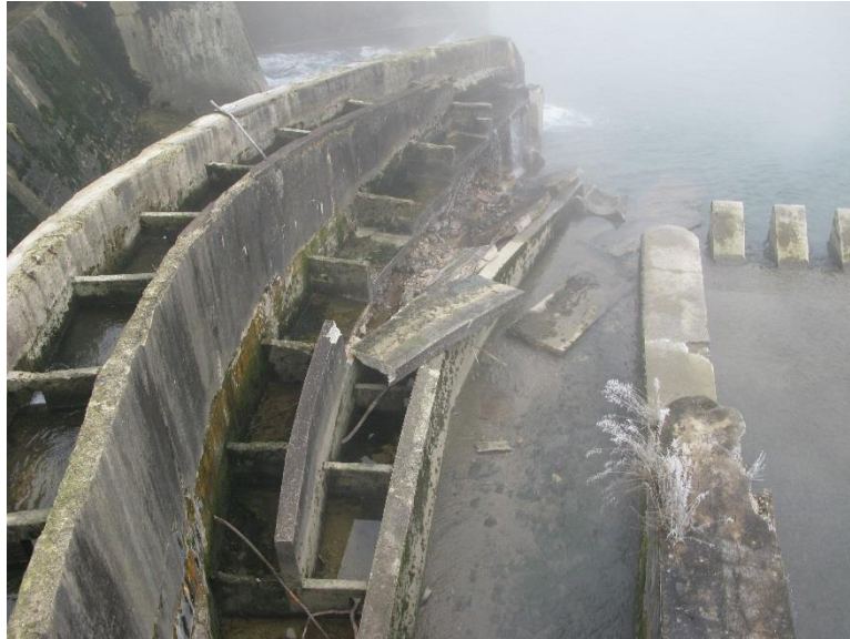
Figure 2: The fish pass at the Fužine weir after its collapse due to high flows
