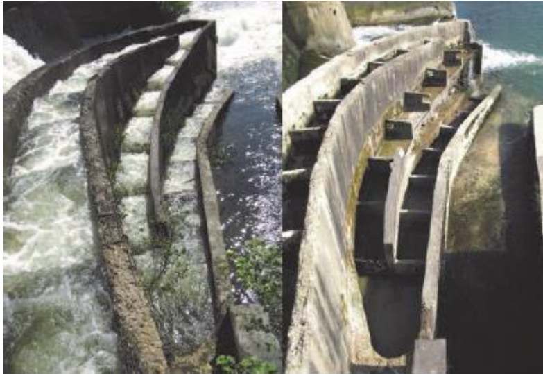
Figure 1: The fish pass at the Fužine weir prior to the restoration and its collapse (left) and after the collapse in autumn 2013 (right).
