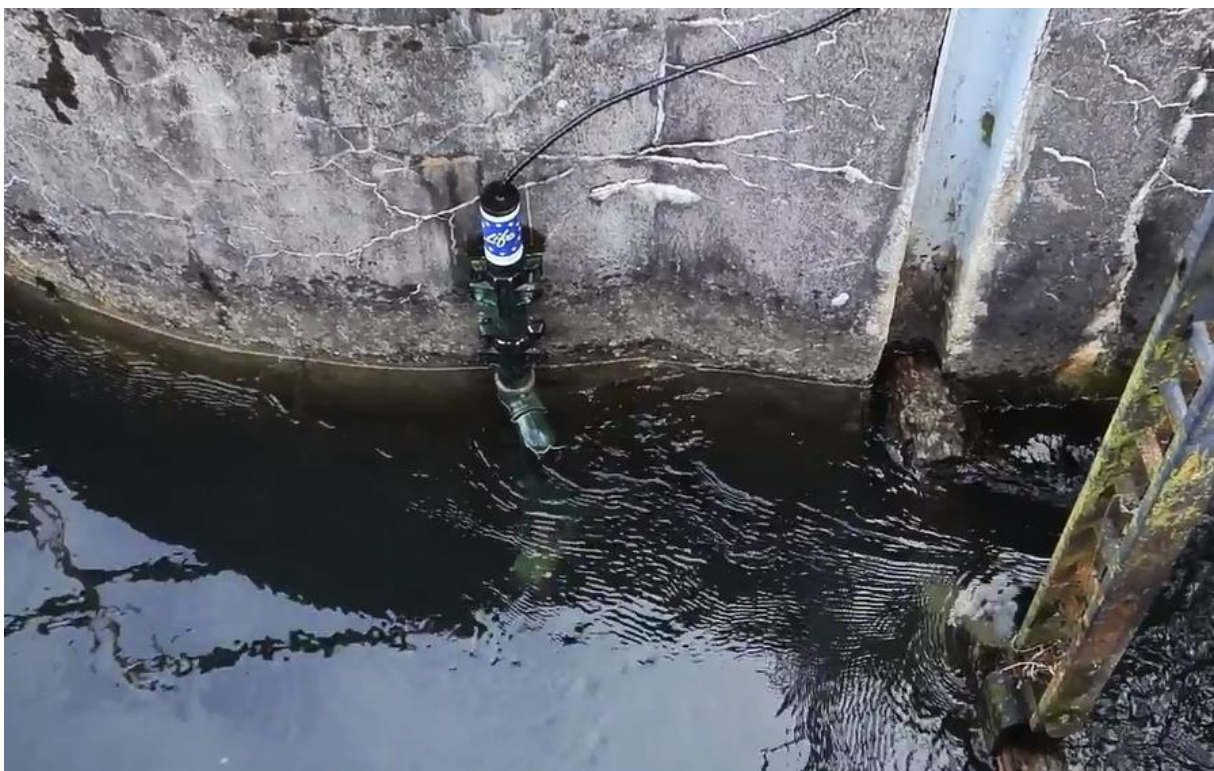
Figure 6: Cameras at the exit of the fish pass at the Fužine weir
