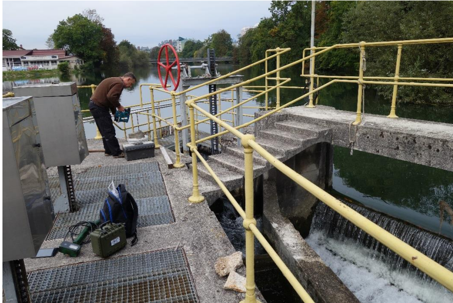
Figure 4: The installation of the cameras following the completion of the works for monitoring the operation of the fish pass
