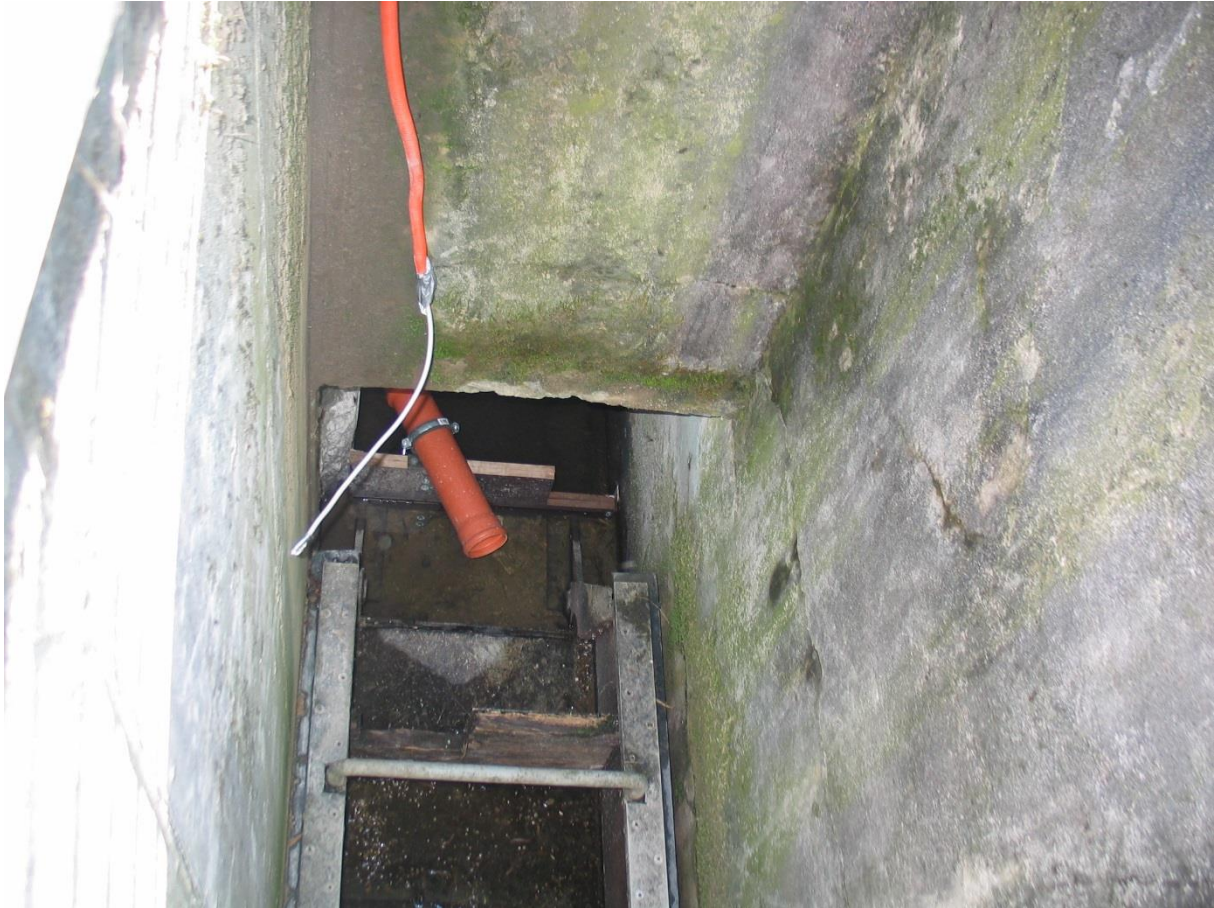
Figure 7: The installation of the attraction pipe and cable on the cable shelf
