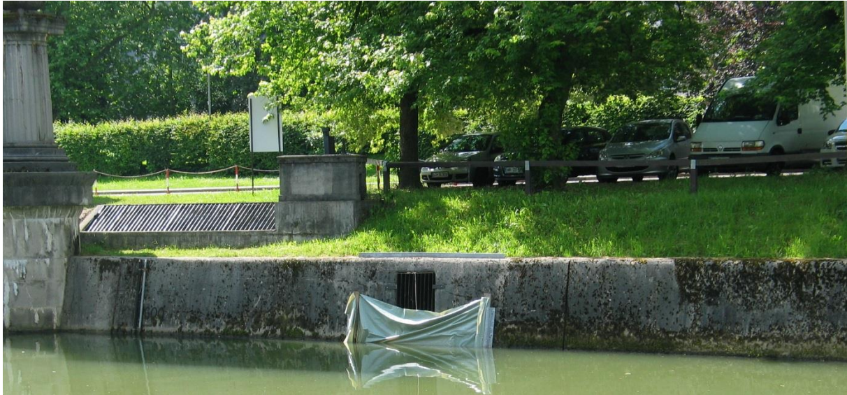
Figure 6: The closing of the fish pass inlet before the start of works inside the fish pass
