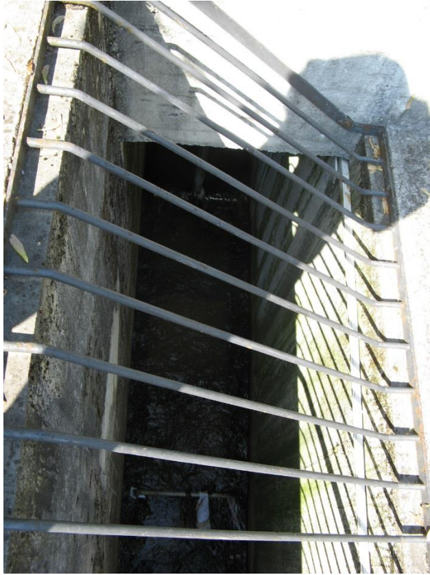
Figure 2: Vertical shaft providing illumination of the fish pass
