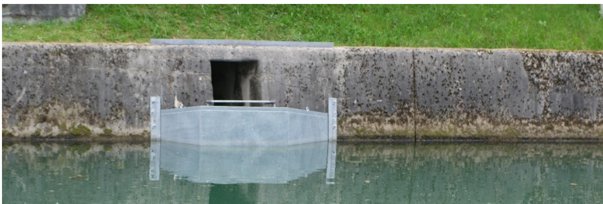
Figure 5: The deflector preventing the debris from flowing into the fish pass
