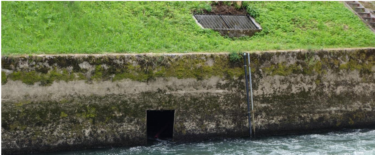
Figure 8: The pipe causing the attraction flow to allow fish to readily locate the entrance to the fish pass
